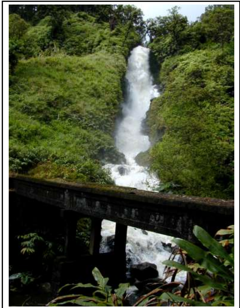
Spreckel's Ditch Overflow, Pu'ohākamoā Stream; RMT CO Bridge (1925) (Photo No. KDA-
