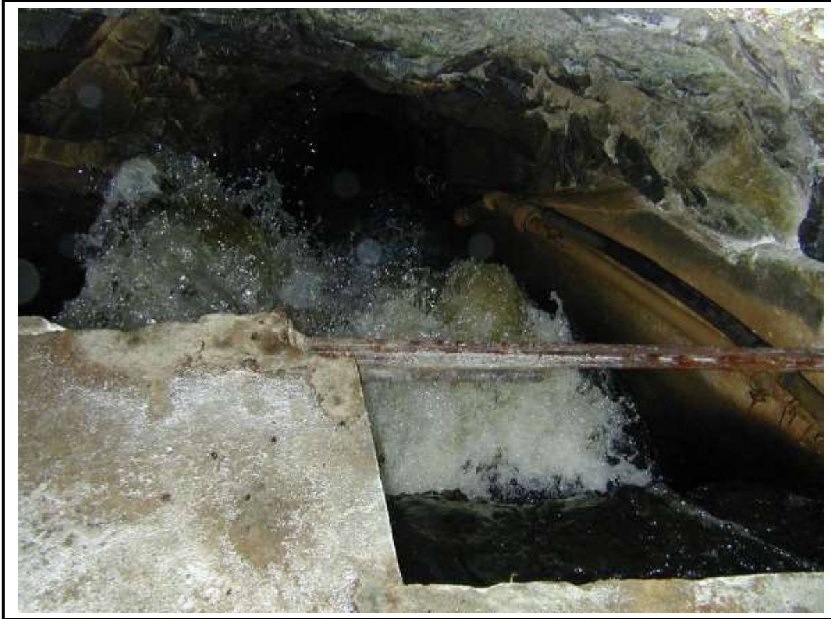
Ko'olau Ditch Tunnel Intake on Pu'ohākamoā Stream (Photo No. KPA-1446)
