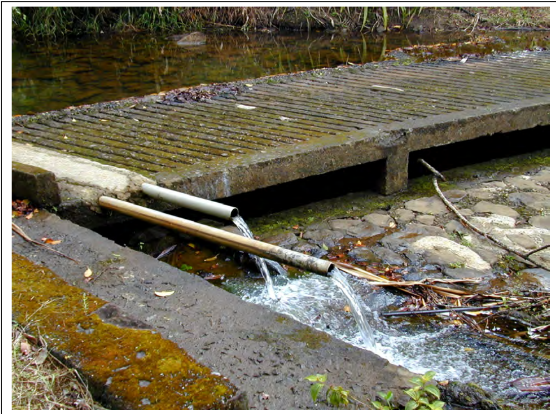
Hai'kū Ditch Intake, Honopou Stream, April 9, 2001 (two pipes drawing water from stream basin for family use); Flow estimated at 200,000 per 24 hour cycle (no rain in preceding day). (KPA Photo No. 1374)
