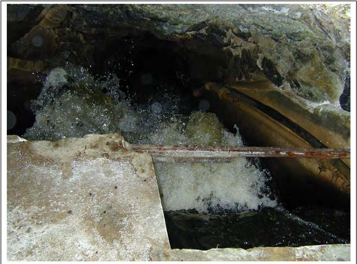
Ko'olau Ditch Tunnel Intake on Pu'ohākamoā Stream (KPA Photo No. 1446)
