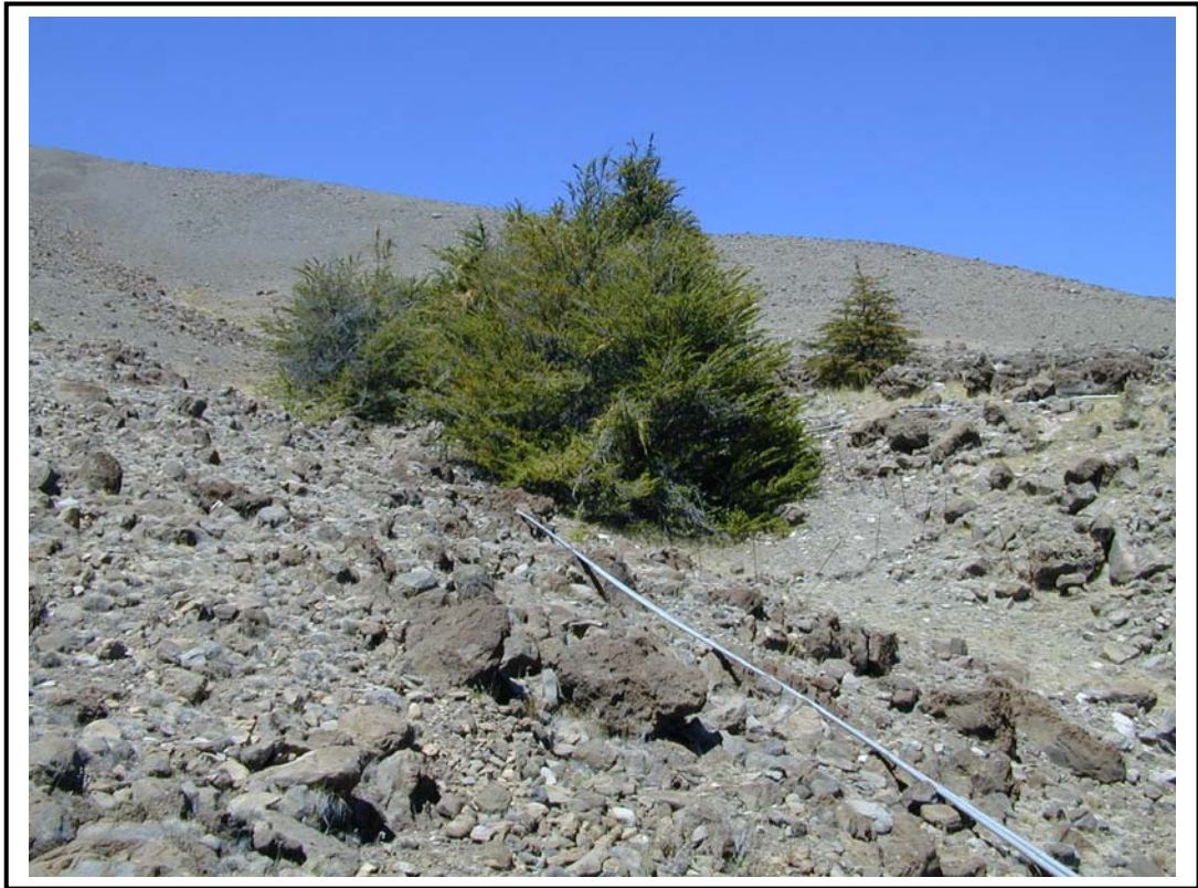
View up to Houpo o Kāne (Hopukani) Spring and present-day pipeline down towards Waihū (Photo No. KPA-N1663)
