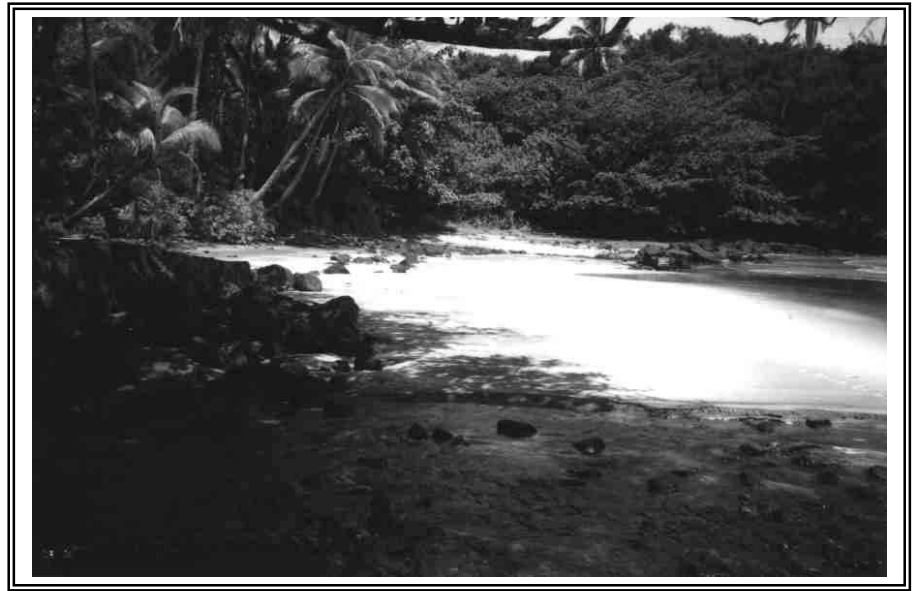
Kea'au Bay – Standing at the outflow of the mākāhā, facing north; partial, single course alignment of stone in sand is a remnant of the Old Government Road. The larger alignment of stones on the water's edge is a remnant of an early 1900s retaining wall built by W.H. Shipman to protect the road and shore line.
