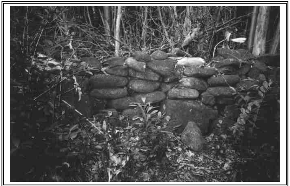
Figure 23. Portion of Stacked Waterworn Stone Wall Site 50-10-36-21263
