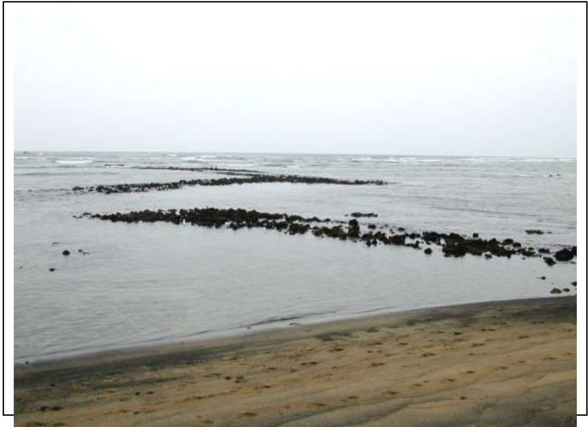
Ruins – Portion of Outer Wall of the Old 'Aimakapā Fishpond (KPA Photo No. 1346)
