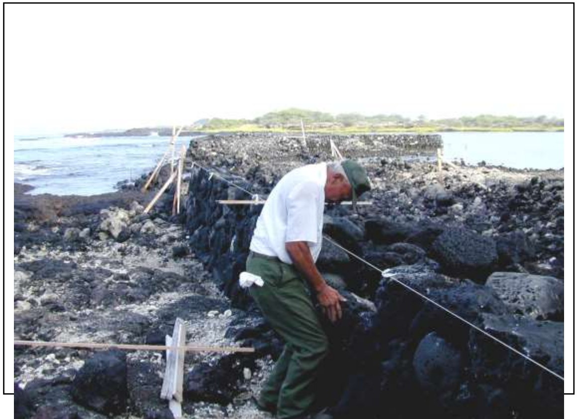
Peter Keka setting Stone in the Pa'ukū (Kuapa) wall of Kaloko Fishpond (KPA Photo No. 1301)
