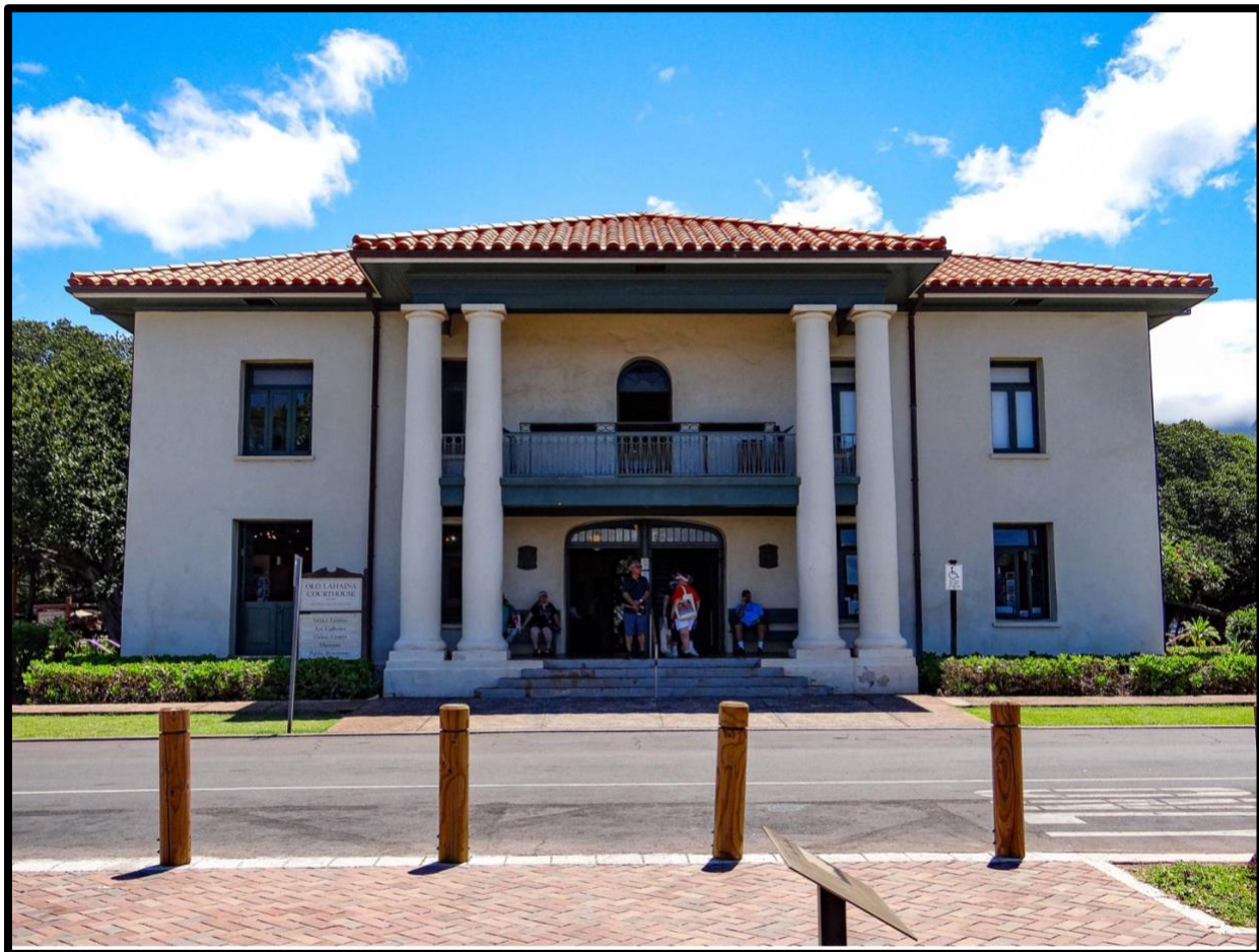
Figure 20. Old Lahaina Courthouse (2022) (Credit: iPhoto Stock Photo ID: 1608989732)
